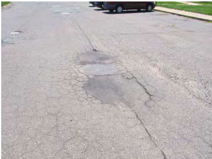
Previous localized repairs have been carried out to the asphalt paved surfaces, however cracking/deterioration is still evident at the present time.
