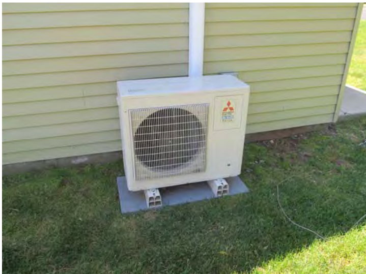
Heating/Cooling needs of Spencer Village Extension are met via ductless, mini-split system heat pumps.
