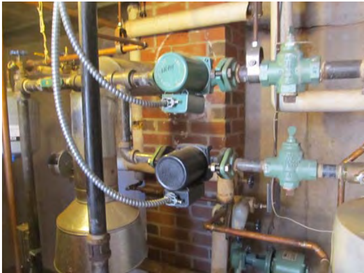
Inline circulation pumps for hydronic heat and domestic hot water.
