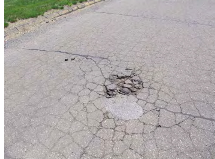
Areas of pot holes were noted within the asphalt paved surfaces.
