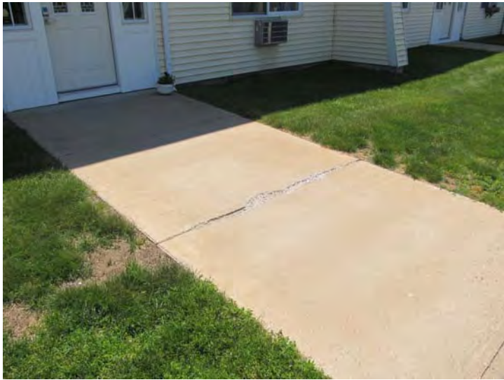
Isolated cracking was noted within the concrete sidewalks.
