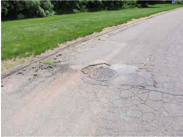
Areas of pattern cracking were noted within the asphalt paved surfaces.
