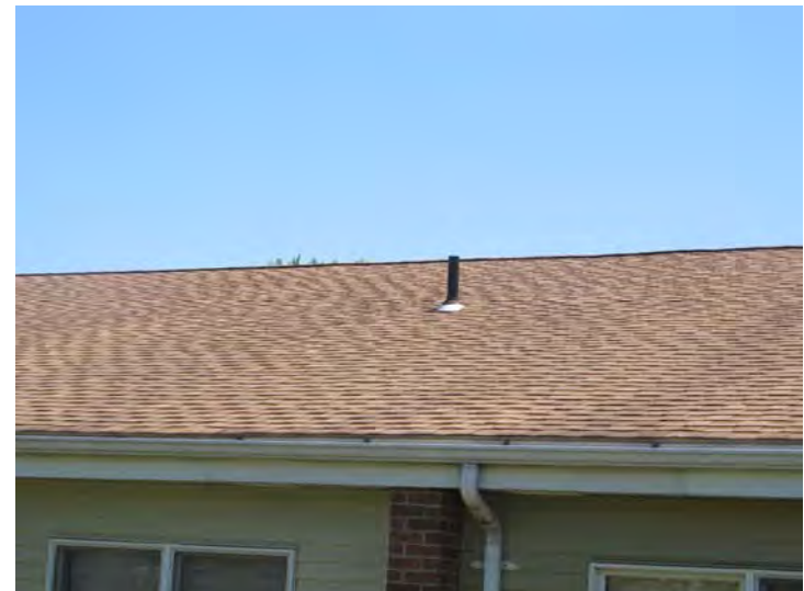
Composite asphalt shingles noted to be in good condition. No widespread deterioration noted.
