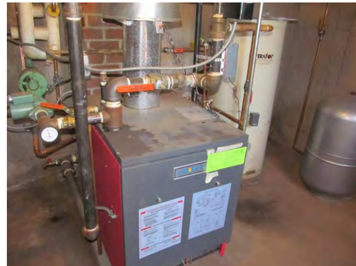
Natural gas fired Crown boiler for production of hydronic heat at Spencer Village.
