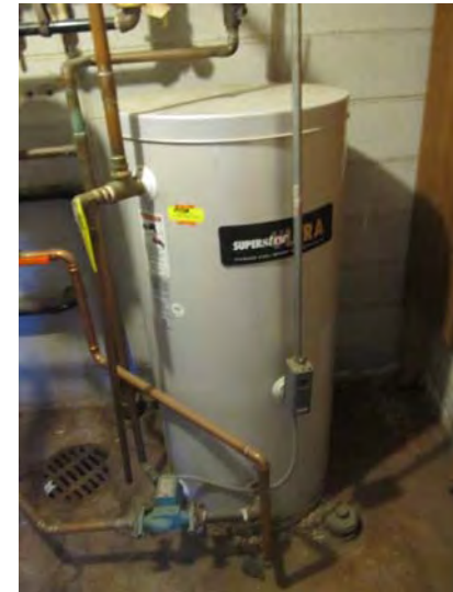
Superstor indirect fired hot water storage tanks of various sizes serve the domestic hot water needs of the original residential development.
